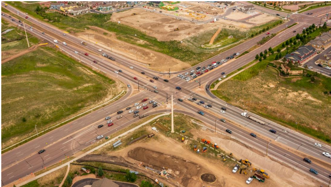
Existing at-grade interchange
